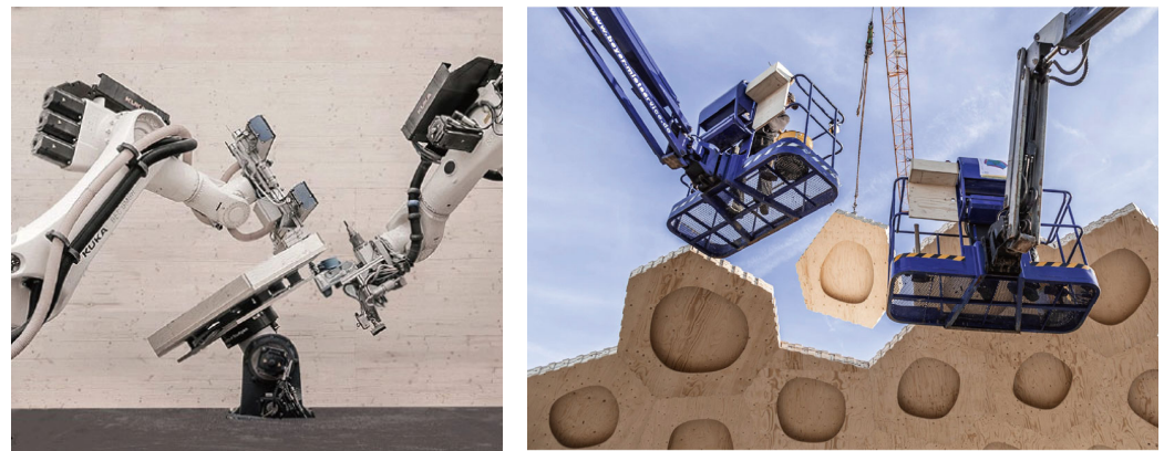
Figure 3. Pre-assembly timber component (left) and on-site assembly of large components (right) © U Stuttgart [37].
